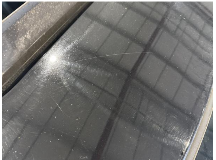
18: Roof Scratched Over 25mm Thru Paint
