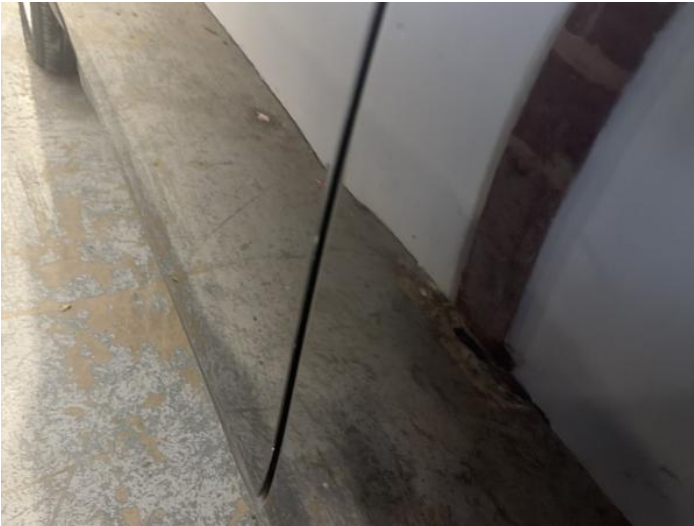
9: Door nsf Chipped Edge Chip
