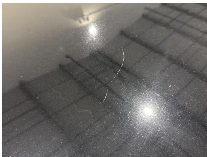
12: Roof Scratched Over 25mm Thru Paint
