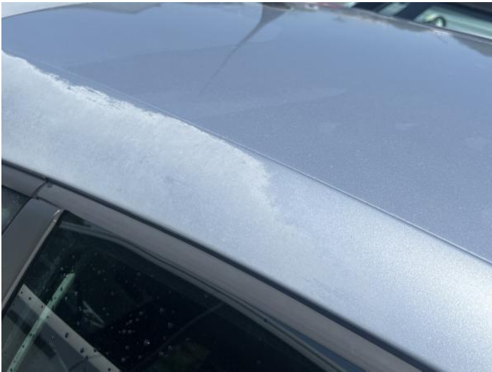
17: C Post os Poor Previous Repair Poor Paint
