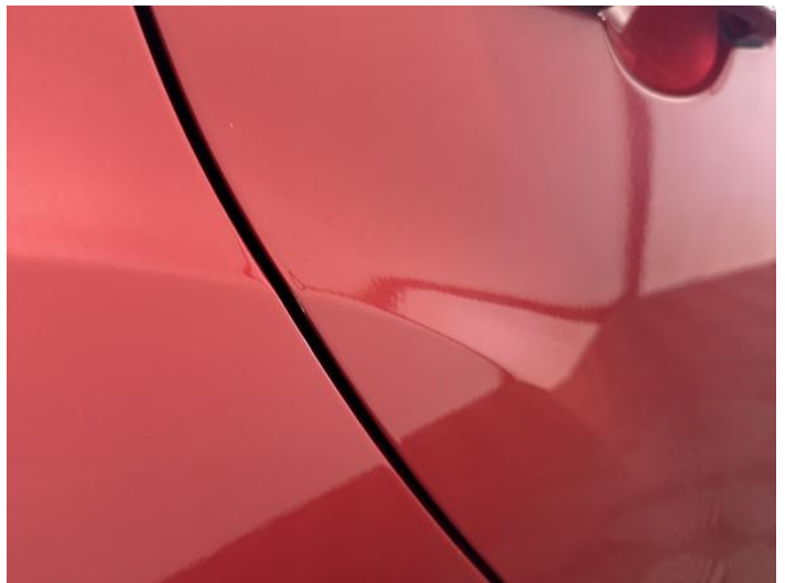
12: Door osf Chipped Edge Chip
