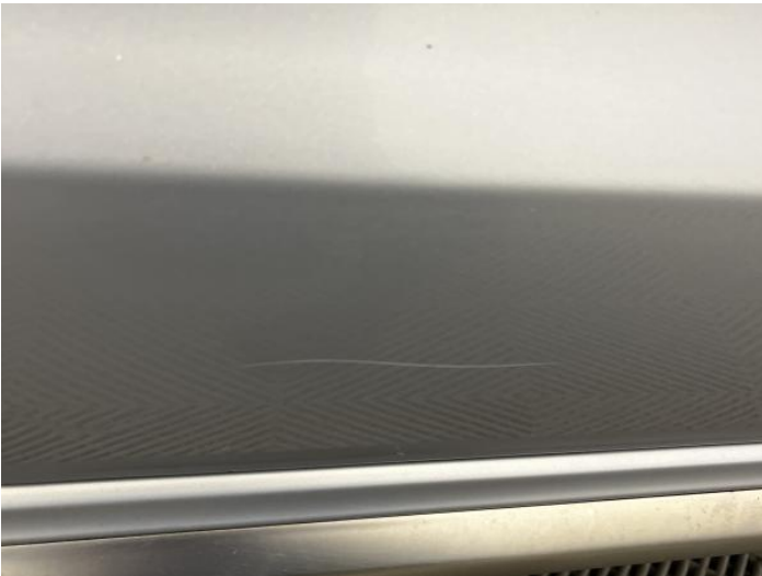
1: Door osf Scratched Over 25mm Not Thru Paint
