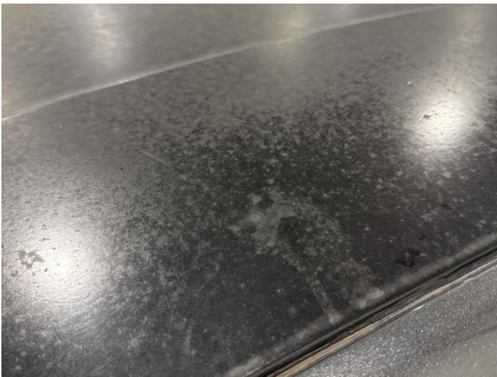
17: Roof Scratched Over 25mm Thru Paint
