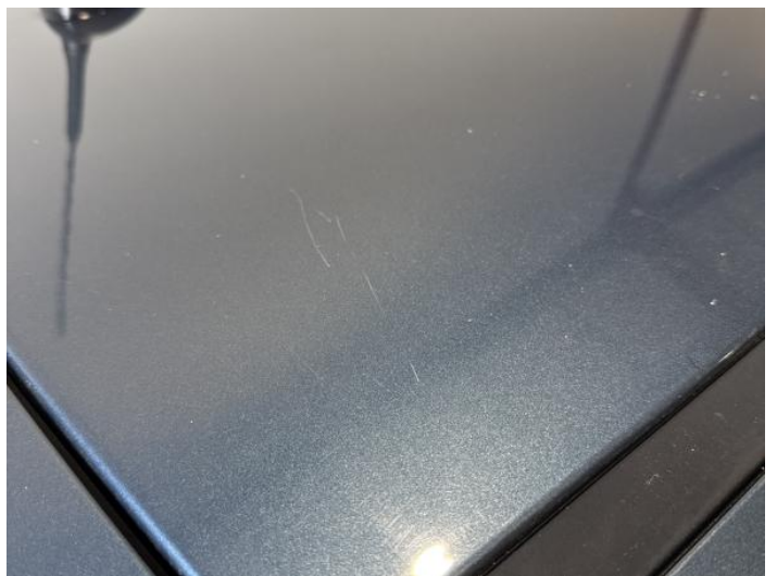
14: Roof Scratched Over 25mm Thru Paint
