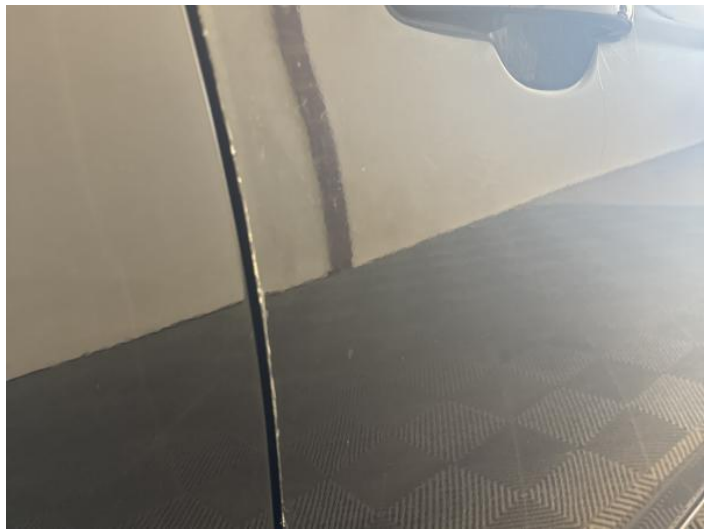
18: Door osf Chipped Edge Chip
