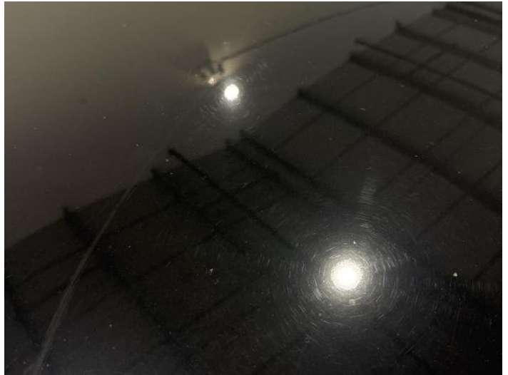
22: Roof Scratched Over 25mm Thru Paint
