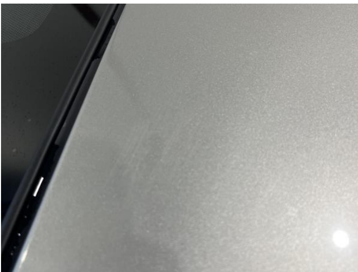
7: Roof Scratched Over 25mm Thru Paint
