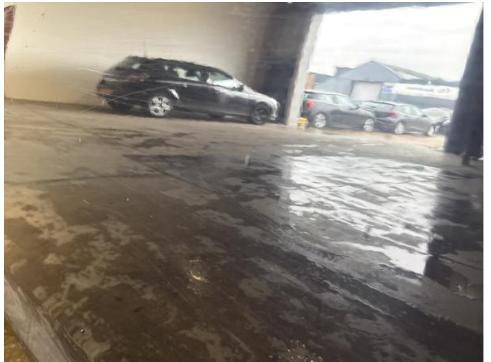
6: Door nsf Scratched Over 25mm Thru Paint
