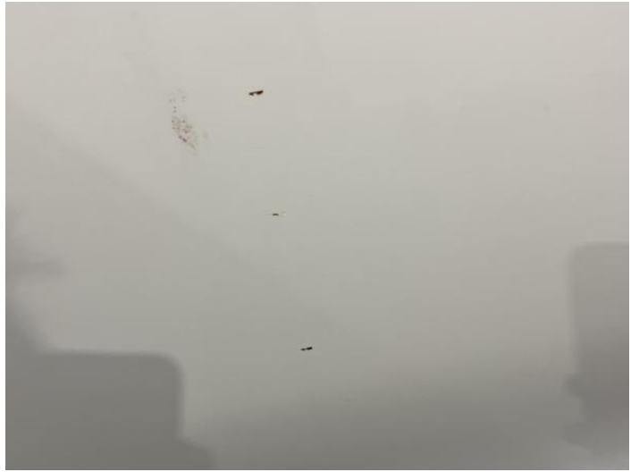
4: Door nsf Scratched Over 25mm Thru Paint
