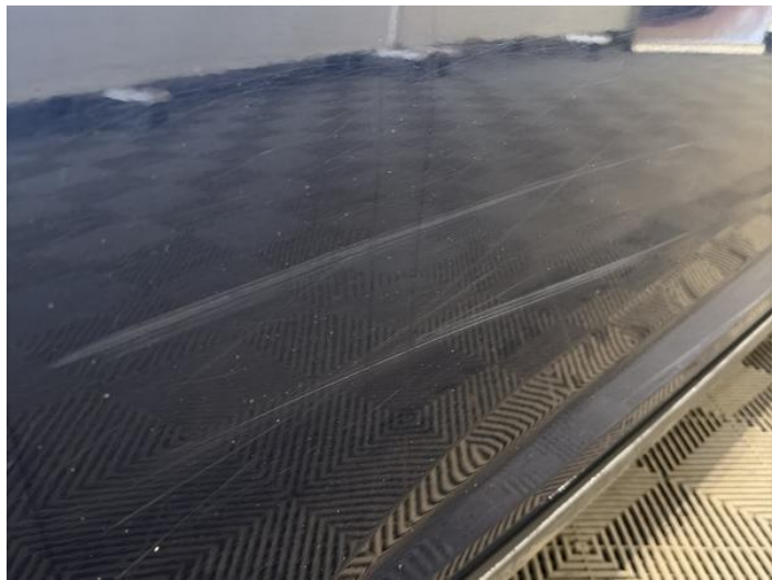
6: Door nsf Scratched Over 25mm Thru Paint
