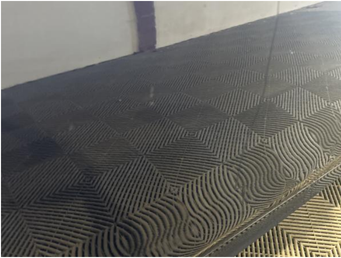
3: Door osf Chipped 1 To 5
