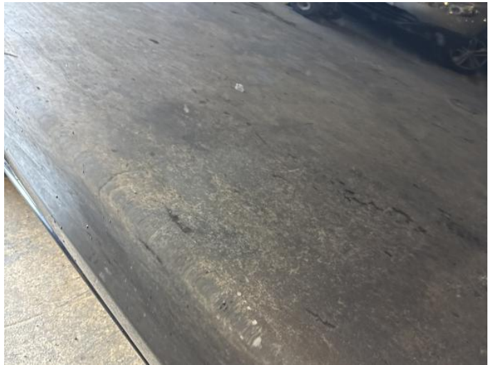
6: Door nsf Chipped 1 To 5
