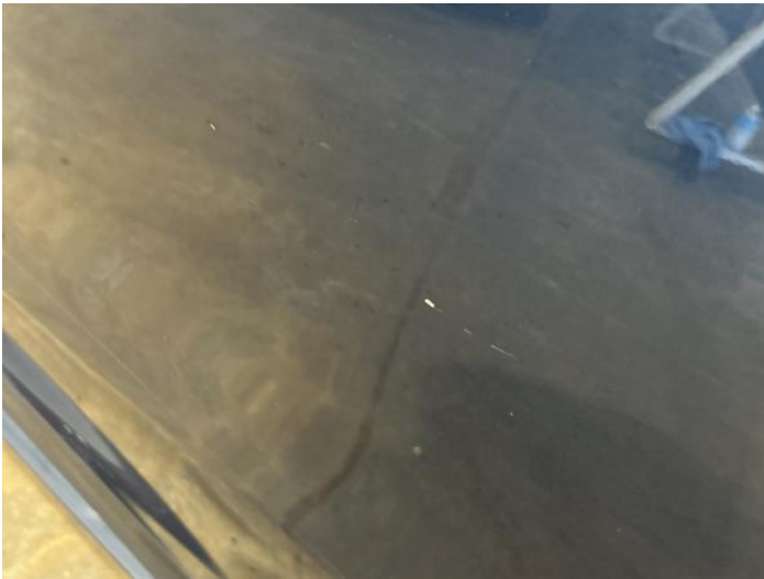
11: Door nsr Chipped 1 To 5
