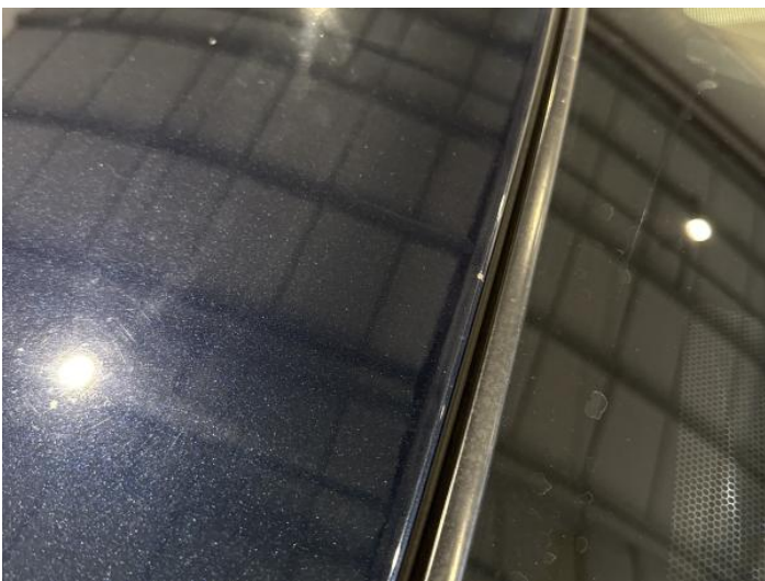
13: Roof Chipped 1 To 5
