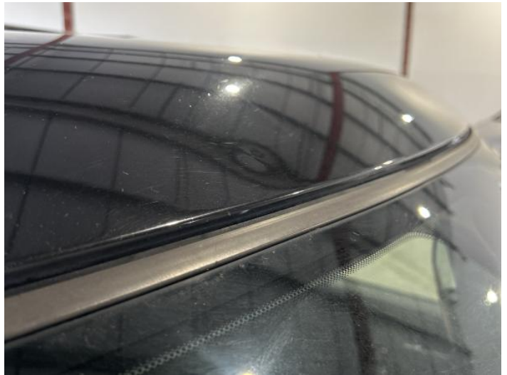
18: Roof Dented Over 30mm
