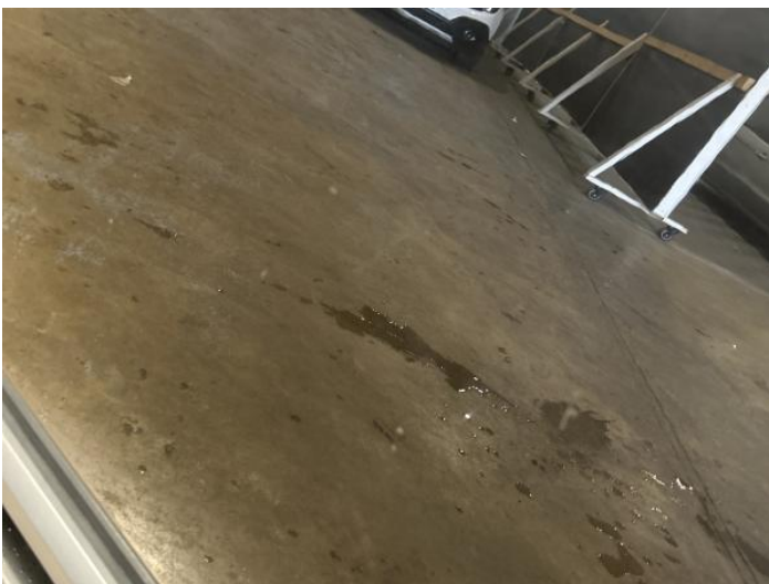
13: Door nsf Chipped 1 To 5
