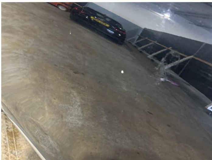
10: Door nsf Chipped 1 To 5
