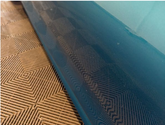
5: Door nsf Dented Between 10mm + 30mm
