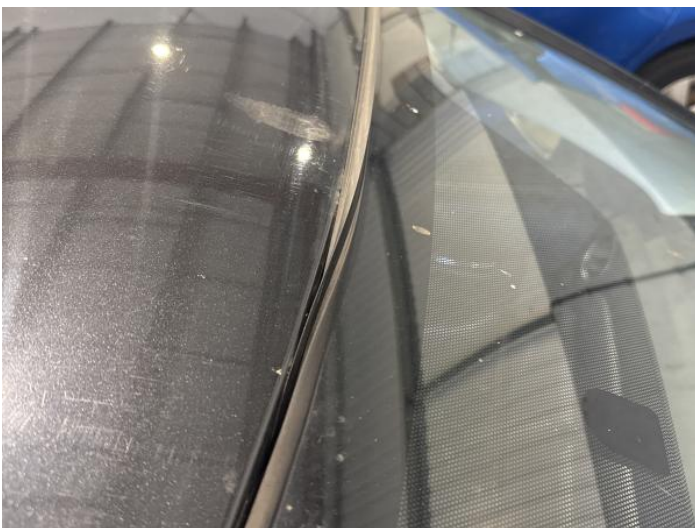
19: Aperture Seal nsf Broken Replace
