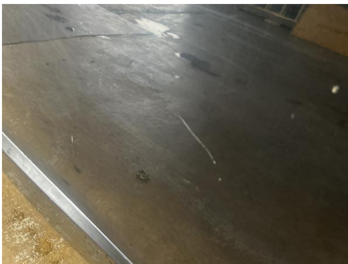
11: Door nsr Scratched Over 25mm Thru Paint
