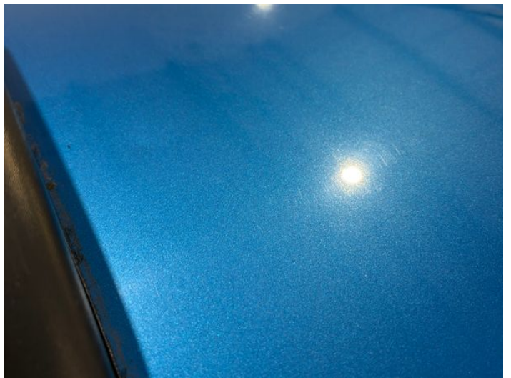
18: Roof Dented Between 10mm + 30mm
