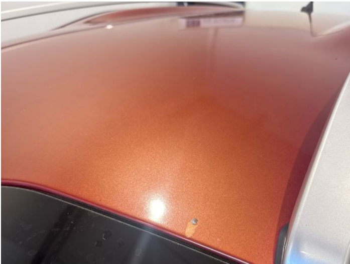
5: Roof Poor Previous Repair Paint Flake
