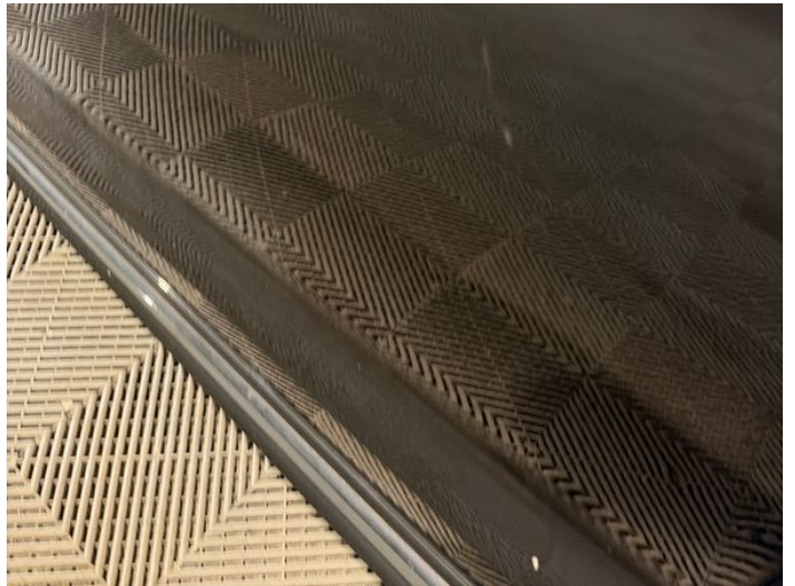
6: Door nsf Scratched Over 25mm Thru Paint
