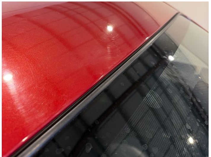
18: Roof Scratched UpTo 25mm Thru Paint
