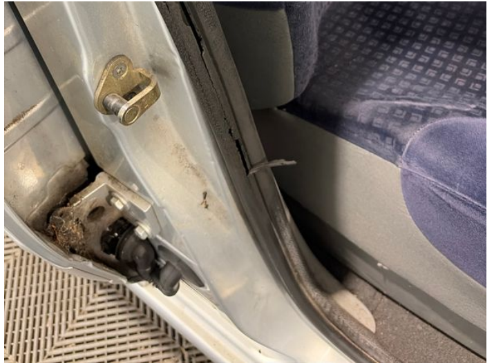
22: Aperture Seal osf Broken Replace
