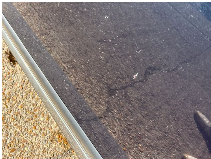
10: Door nsf Chipped 1 To 5
