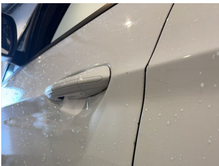
5: Door nsf Chipped Edge Chip
