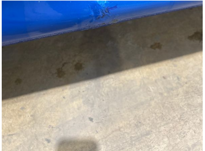
4: Sill os Rusted Over 5mm
