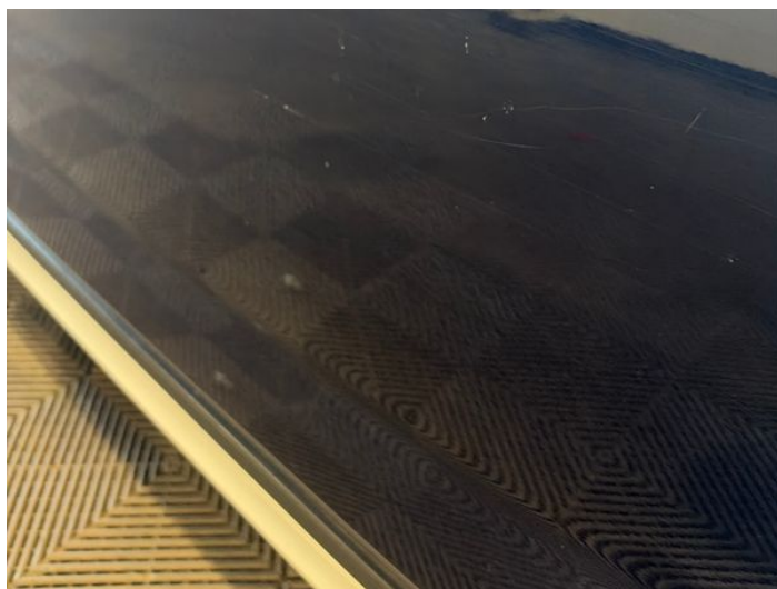
6: Door nsf Scratched Over 25mm Thru Paint
