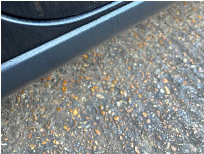
18: Door osf Rusted UpTo 5mm
