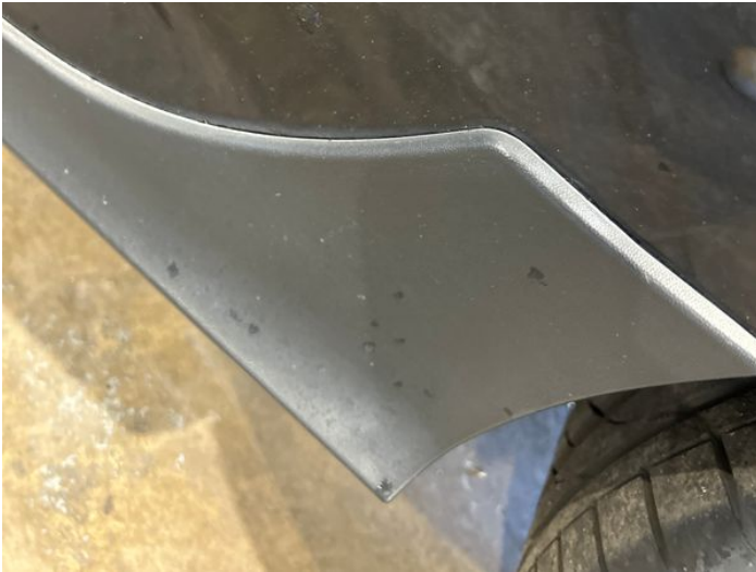
9: Qtr Panel nsr Rusted Over 5mm
