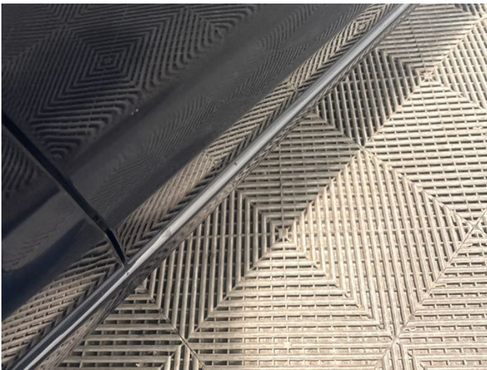
17: Door osf Chipped 1 To 5
