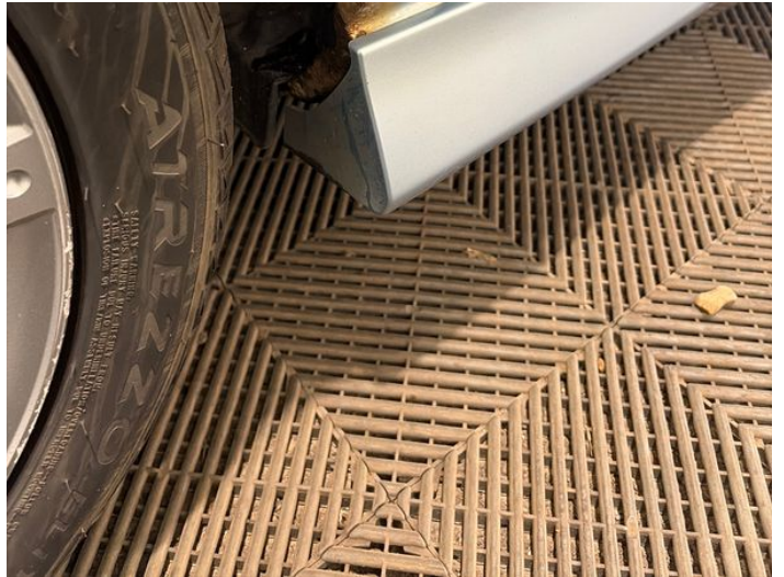
16: Sill os Rusted Over 5mm
