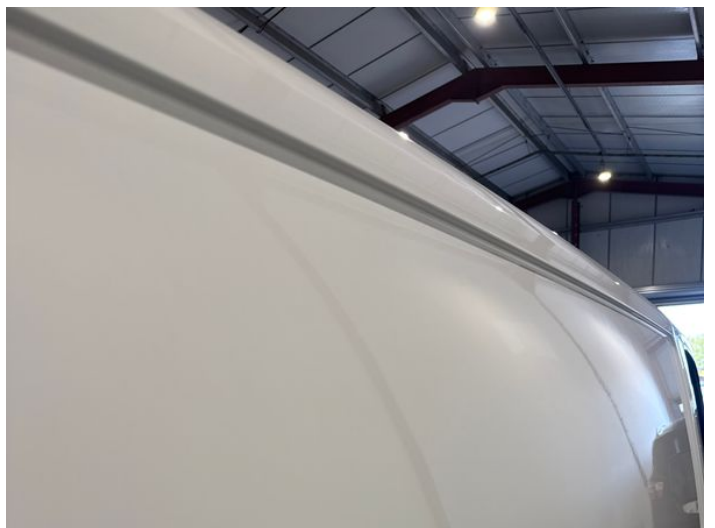
14: Qtr Panel osr Dented Over 30mm
