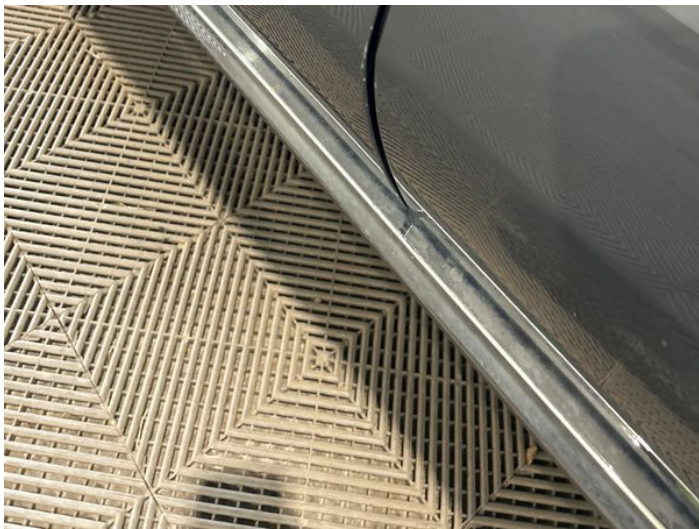
9: Door nsf Chipped Edge Chip
