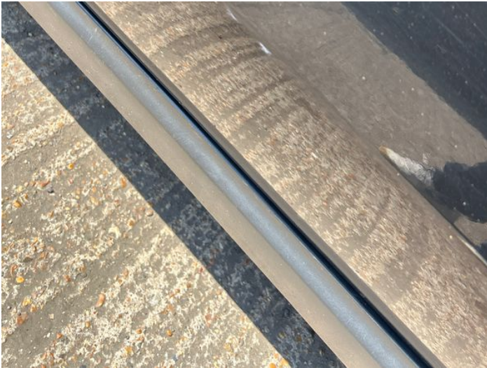
3: Door osf Chipped 1 To 5
