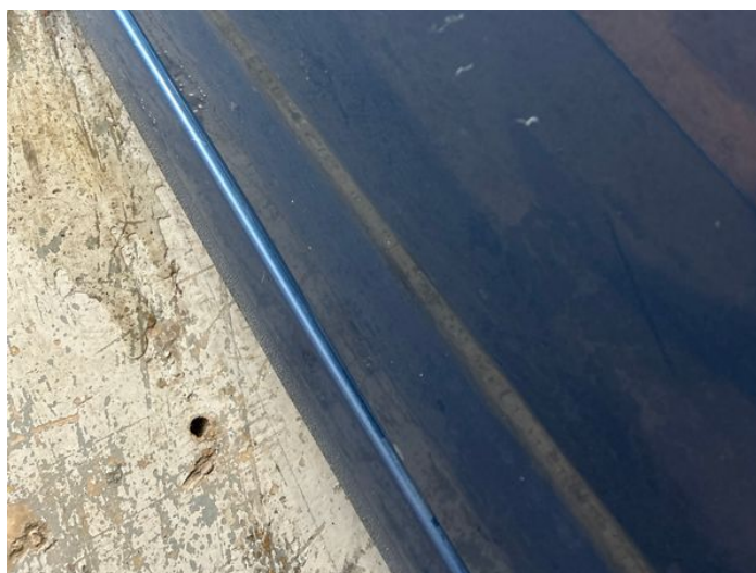
8: Door nsf Chipped Multiple Chips
