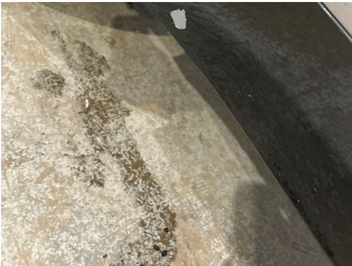
13: Door Moulding osr Scratched (Painted) Over 25mm Thru Paint
