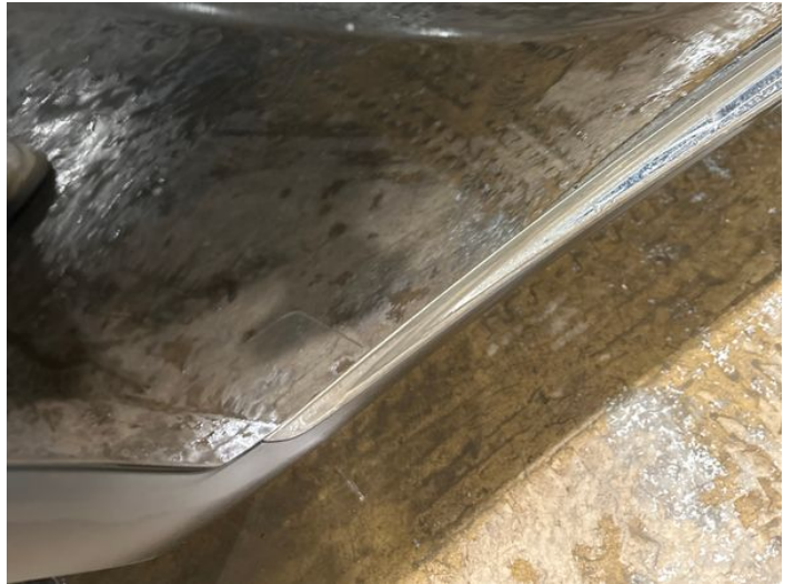
10: Door osr Chipped 1 To 5
