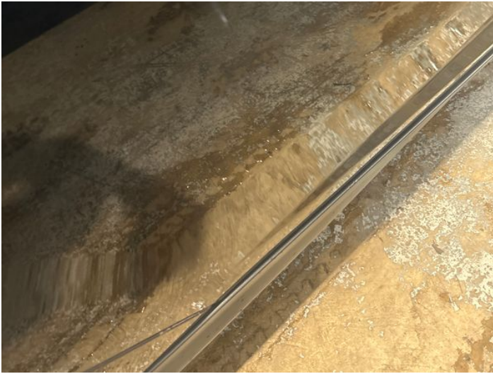
3: Door osf Scratched UpTo 25mm Thru Paint
