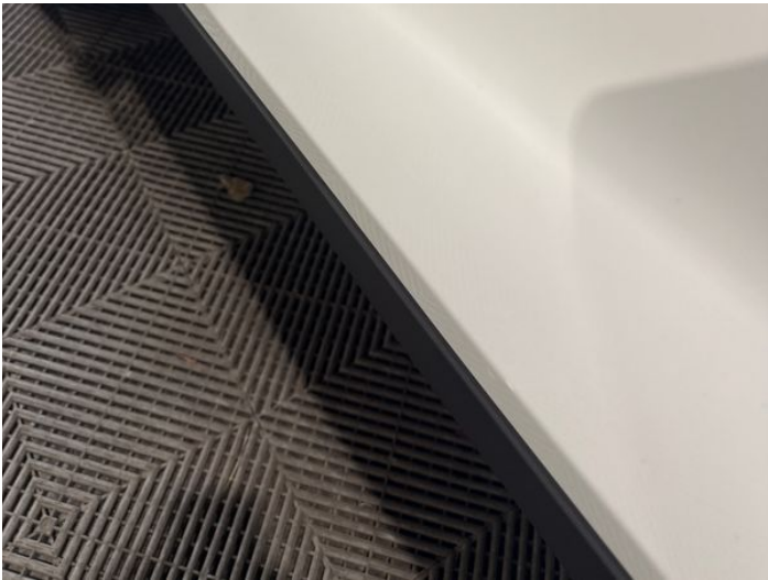
5: Door nsf Dented Over 30mm
