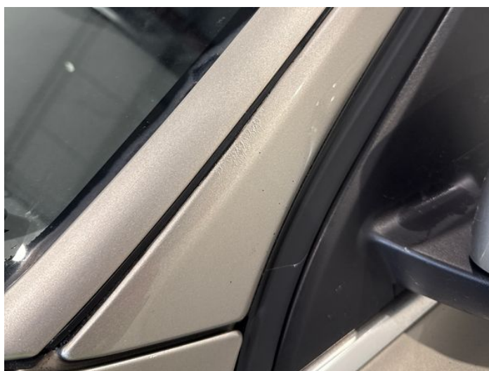
6: A Post ns Rusted Over 5mm
