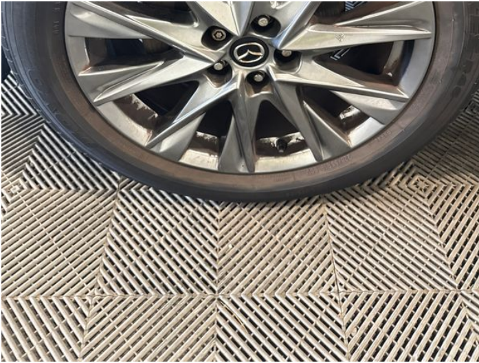
3: Wheel nsf Corroded Light
