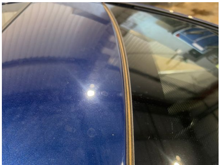
8: Roof Chipped 1 To 5
