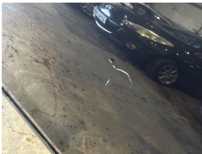
2: Door osf Scratched Over 25mm Thru Paint
