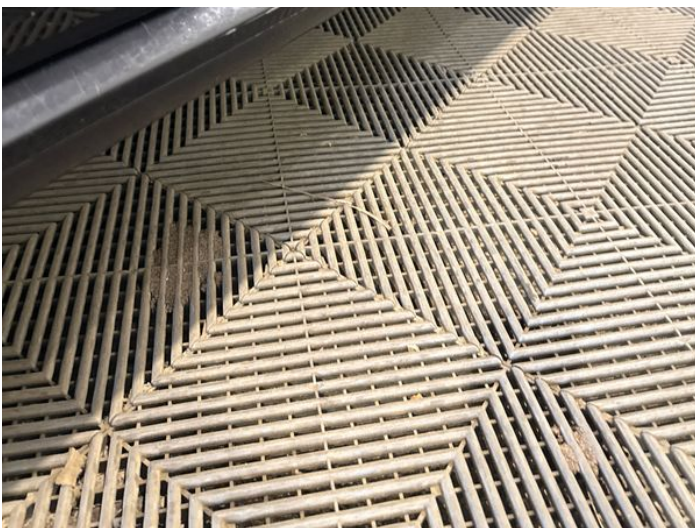
7: Sill ns Scratched Over 25mm Thru Paint
