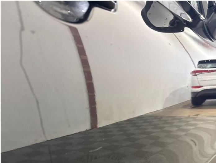
15: Door osf Scratched UpTo 25mm Thru Paint
