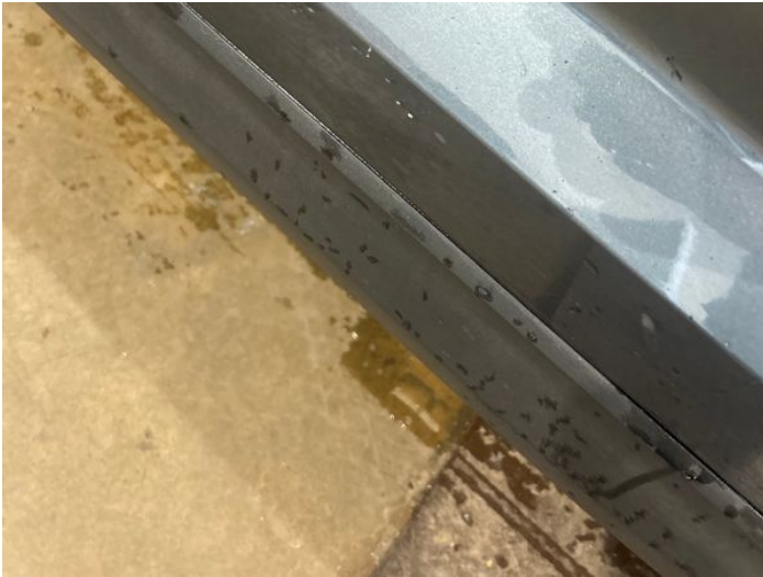
3: Door osf Chipped 1 To 5
