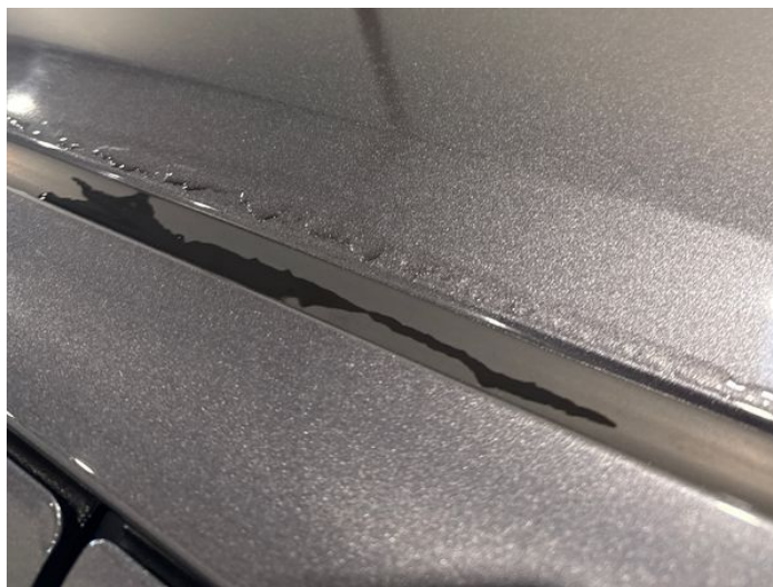
2: Roof Dented Between 10mm + 30mm
